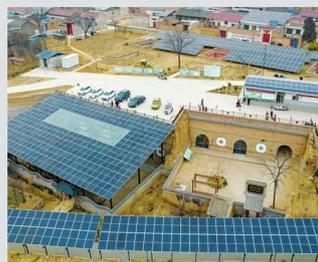
The Zero Emission Village in Zhuangshang, Shanxi province, is a model project to deploy distributed PV and energy storage in rural areas. With a total installed capacity of 2 MW, many of the village’s households are now equipped with solar panels, energy storage, and smart inverters and can both supply power to the rest of the village and sell surplus electricity to the country’s main grid company, State Grid Corporation of China.
