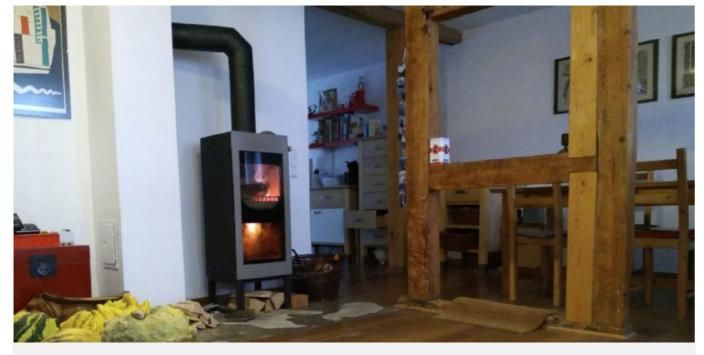
A typical application is this stove in a private single-family house (with a living space of 170 m2). The stove covers approximately 30% of the heat demand of the building. The rest is covered by a conven-tional heating system. The wood is delivered by a local biomass supplier and partly covered by private wood supplies. Essential for the twin-fire operation is dry and clean wood and an adequate ignition process of approximately 20 min.
