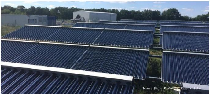
Since 2016, the largest German solar thermal installation has been in operation in Senftenberg (24,000 inhabitants). By means of 8,300 m<sup>2</sup> of ETC-collectors, 4% of the yearly heat demand of the district heating system is provided by solar energy, replacing an equivalent amount of heat from a lignite power plant. The system uses no storage at all. The temperatures in
