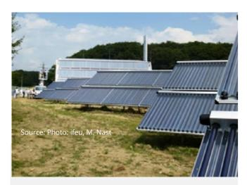
The first commercial collector field to feed heat into a district heating network was installed in 2012 in Büsingen, a village with 1,300 inhabitants. Through about 1,000 m<sup>2</sup> of ETC collectors and a heat storage tank (100 m<sup>3</sup>) 12% of the heat demand of the network is covered by solar energy. The remaining part is provided by two wood chip boilers. 107 oil boilers in private and public buildings were substituted with the renewable district heating system.
