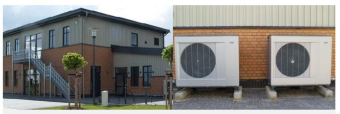
The fire station was built is 2014. Two air source heat pumps were installed for space heating and for domestic hot water. The heat is distributed through panel heating in the rooms. The rooms are supplied with three different temperature levels, which depend on the use schedule and the activities to be performed. There are PV modules on the roof to supply the accumulator, which is used to se-cure the electricity supply during blackouts. Source: [1]
